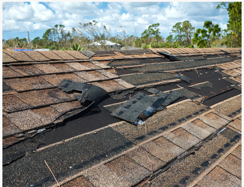
Post Hurricane Roof Damage
