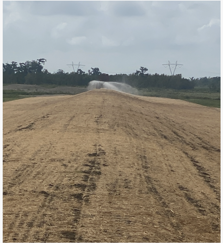
Once the levee is cleared, seed is spread and watered to promote a stronger levee.
