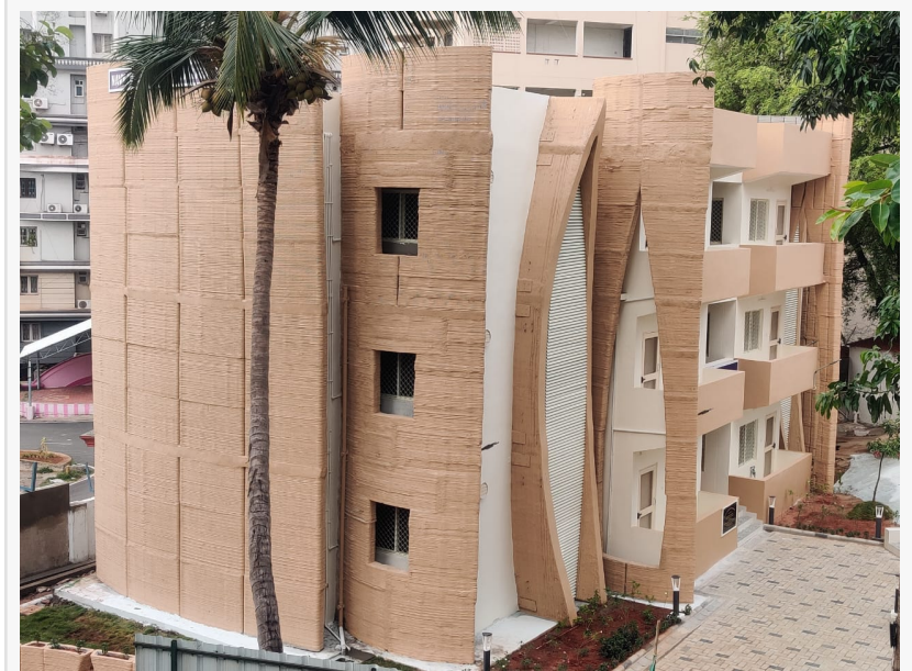
MiCoB 3D Printed Building for Indian Navy
