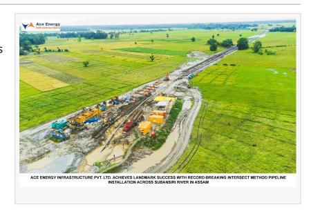
possible by utilizing the intersect method of Horizontal Directional Drilling (HDD), positioning it among the largest pipeline installations worldwide using this technique.
