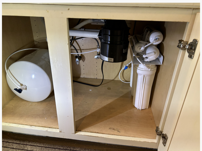
Installation of reverse osmosis
