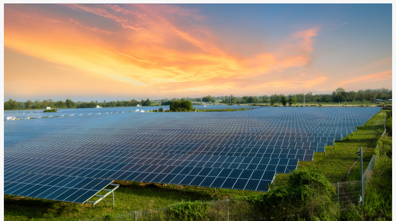
REPOWER Orange installs high-efficiency commercial solar panels in Orange County, California
