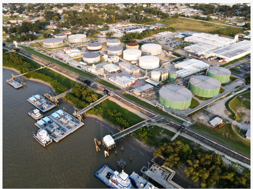
Stone Oil's Gretna, Louisiana, facility
