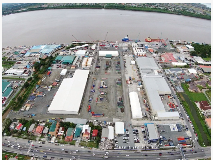
TOTALTEC Inc located in proximity to Guyana Shore Base Inc
