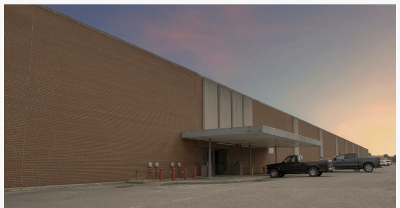
ReElement Technologies Marion Indiana Facility
