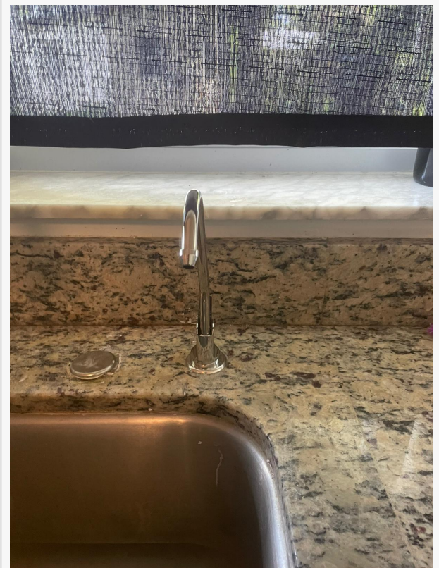
Installation of faucet for R.O
