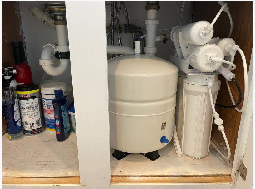
reverse osmosis install
