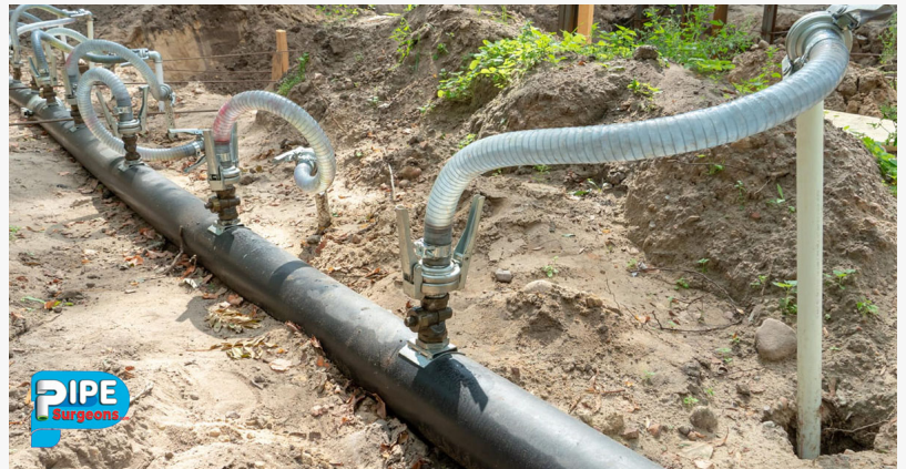
Pipe Repair Service in Vero Beach
