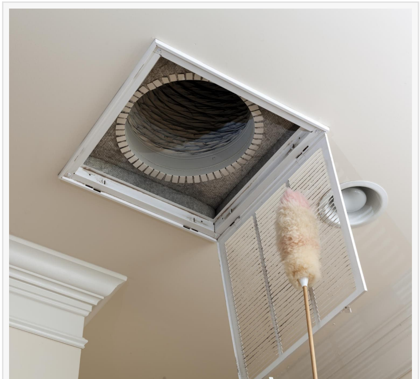
Air Duct Cleaning Services
