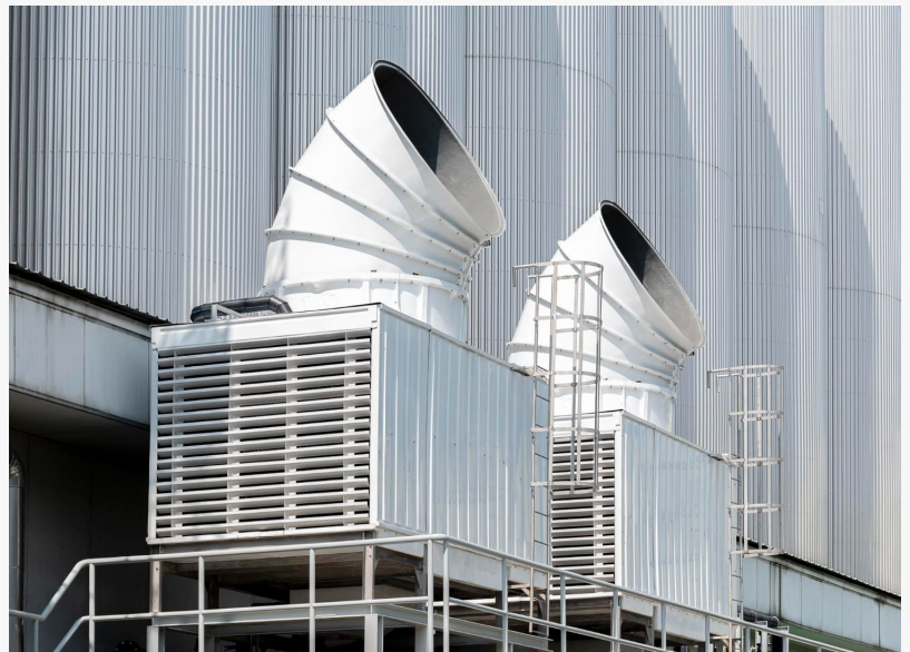
Air Duct Cleaning Service PSL
