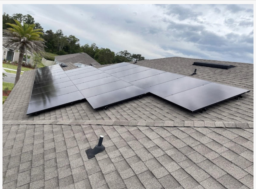
Recent Solar Panel Installation
