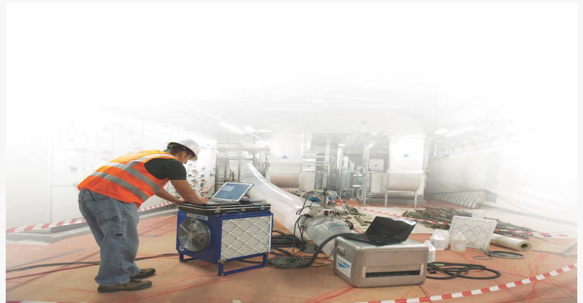
An Aeroseal worker seals a commercial building's air ducts with the company's patented technology.
