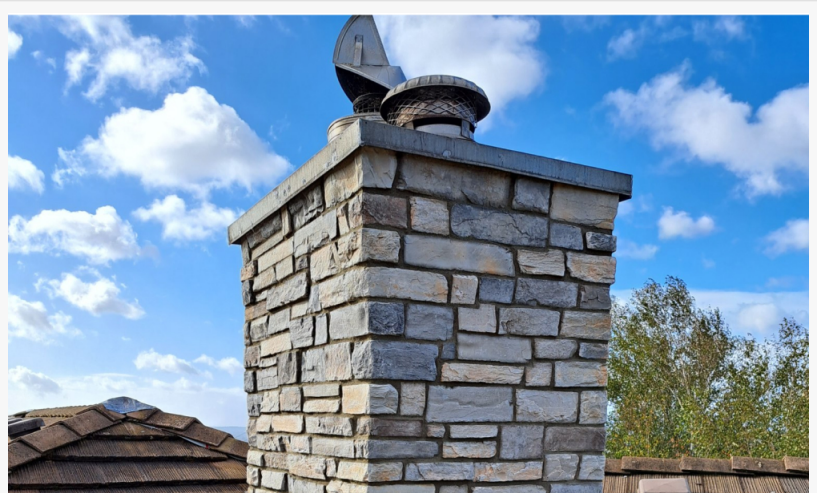
Stone Masonry Chimney Installation and Repair
