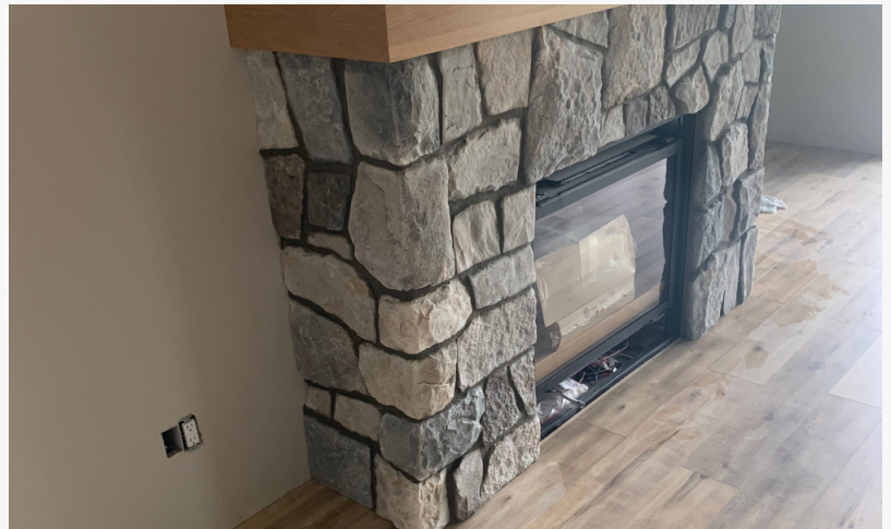
Stone Masonry Fireplace Installation and Repair
