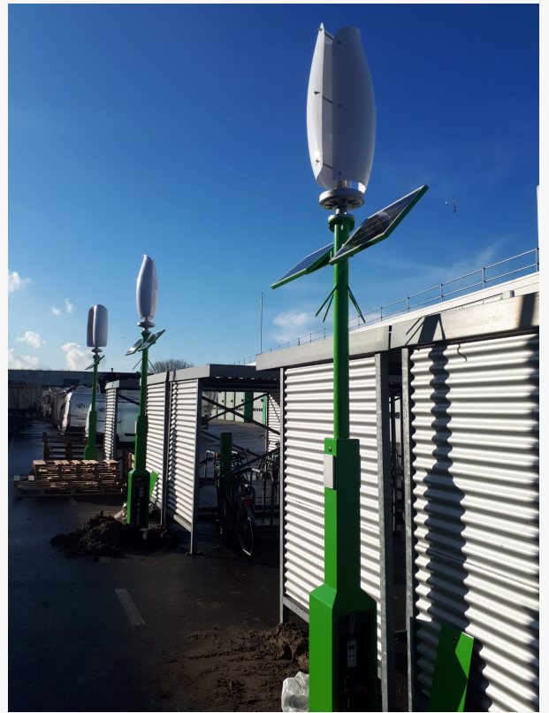
Wind and Solar E-bike Charging Poles
