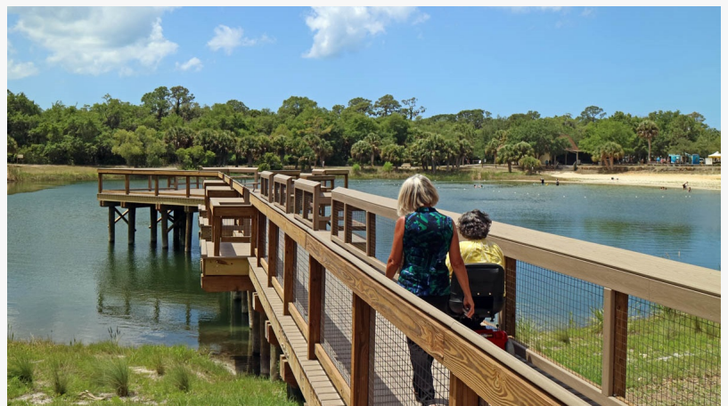
An accessible pier at Oscar Scherer State Park offers areas of lowered rails so that seated visitors have unobstructed views and may cast fishing lines.
