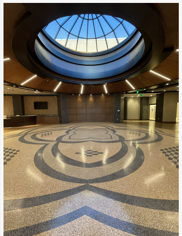
Traditional basketry patterns inspired the award-winning terrazzo floors installed in the Agua Caliente Resort Casino & Cultural Museum.
