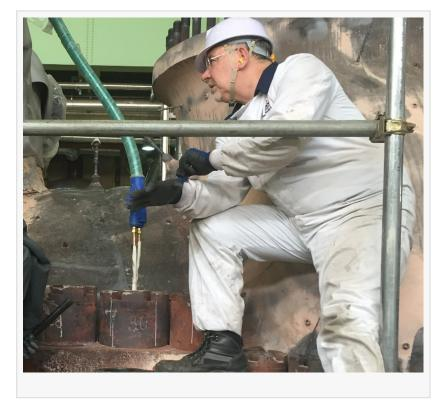
Induction heating, Thermo International's specialty, is a process that utilizes the electrical conductivity of metals to heat materials rapidly and precisely with an electromagnetic field produced by a coil. Thermo specially designs these coils to work with our portable induction equipment for this and a range of additional applications.
