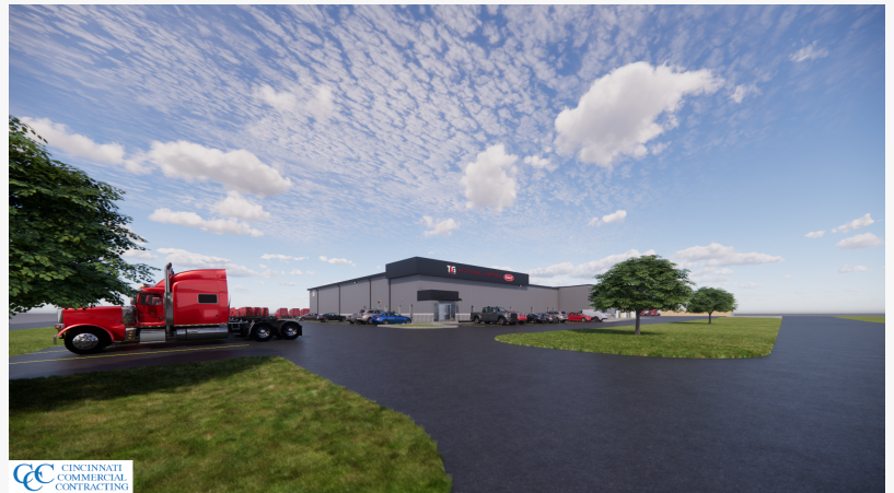
The upgrades and expansion at TLG Peterbilt - Evansville are slated to be completed Fall 2023.
