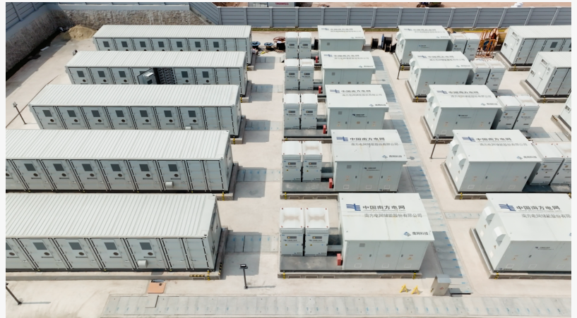
The power station is the world's first to deploy entirely immersion liquid-cooling BESS, using Hithium's technology
