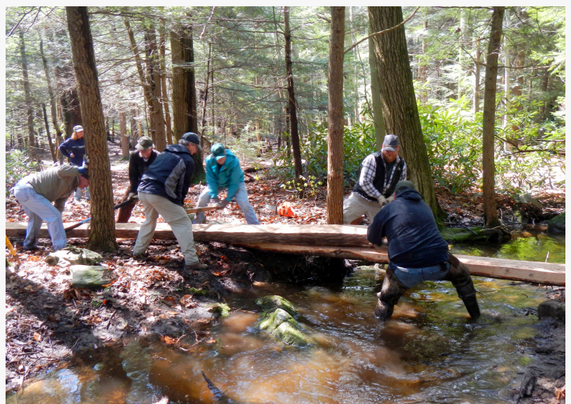
Laurel Ridge State Park volunteers help build a trail bridge
