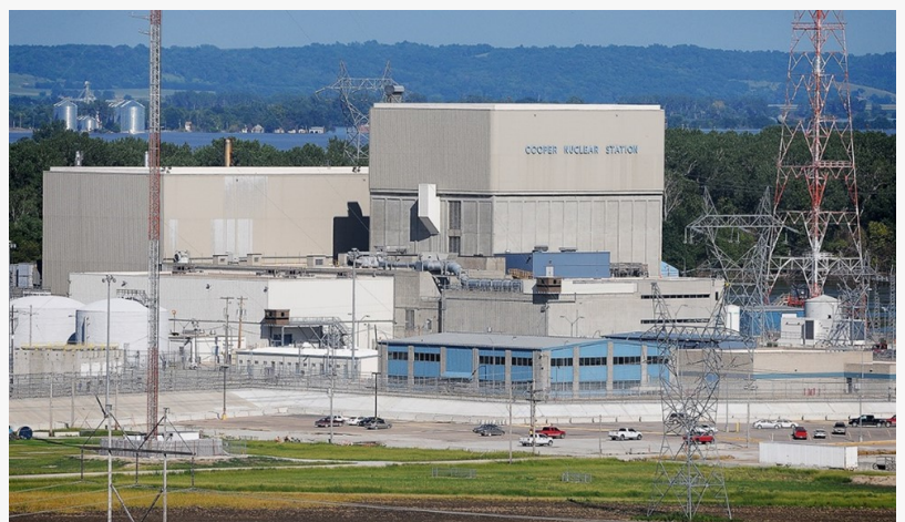
Cooper Nuclear Station (Source: NPPD)
