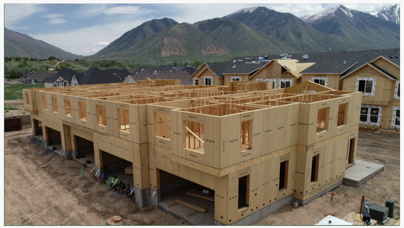
BamCore Prime Wall™ Framing System at the Concord Homes, River Run, Multi-Family in Utah
