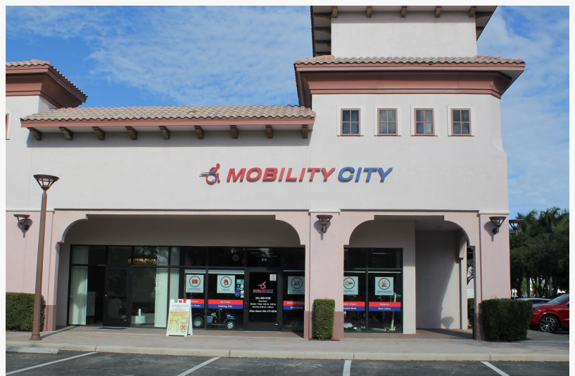
Mobility City Headquarters and Showroom, 1200 Yamato RD, A9, Boca Raton, FL 33431
