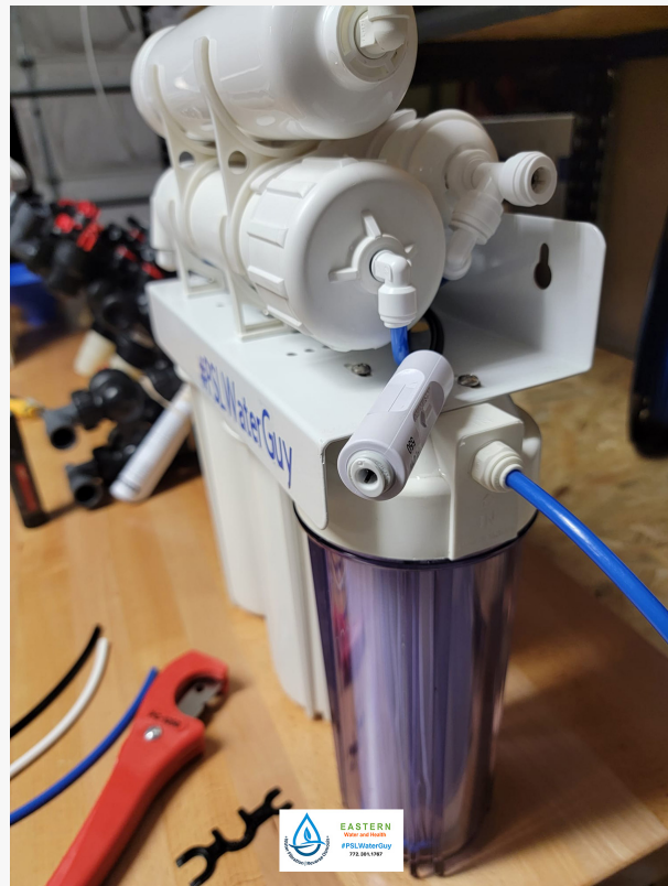
Under-the-Sink Reverse Osmosis Installation
