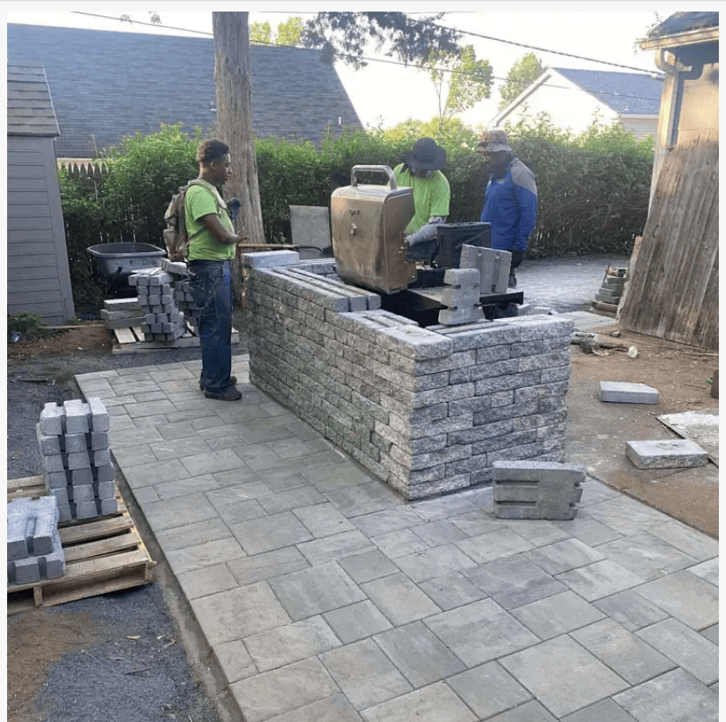
Outdoor Kitchen Build & Installation
