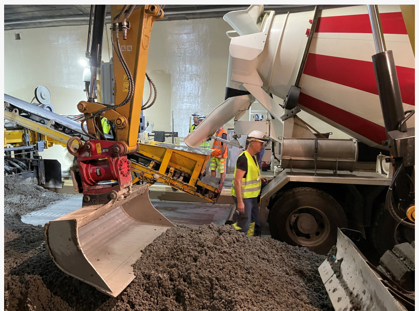
Workers in the Arlbergtunnel monitored by Crew Companion
