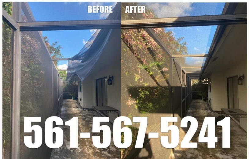
iRepairScreenPatios Work Sample 2 (Before & After)
