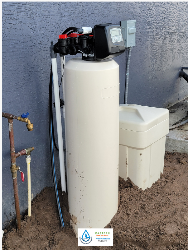
Water Softener System Installation Port St. Lucie
