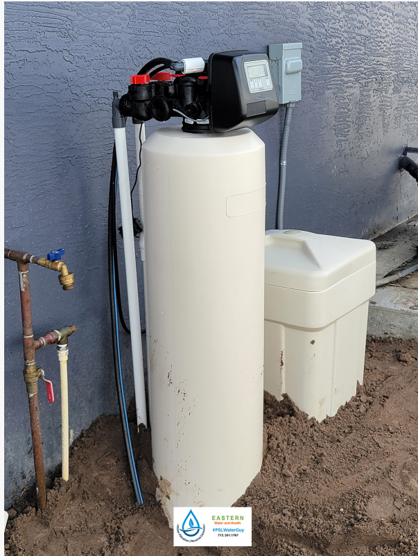
Water Softener System Installation St. Lucie County
