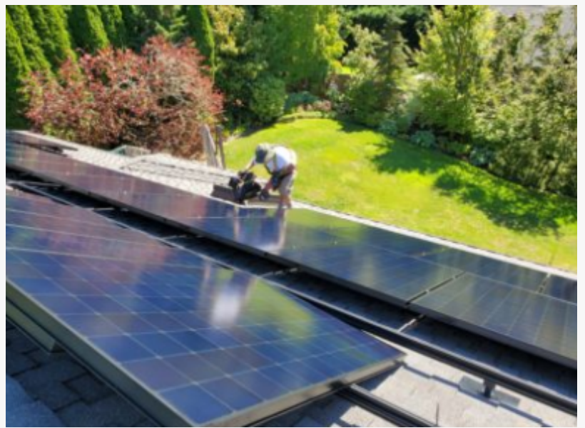
Sunergy Systems Installation
