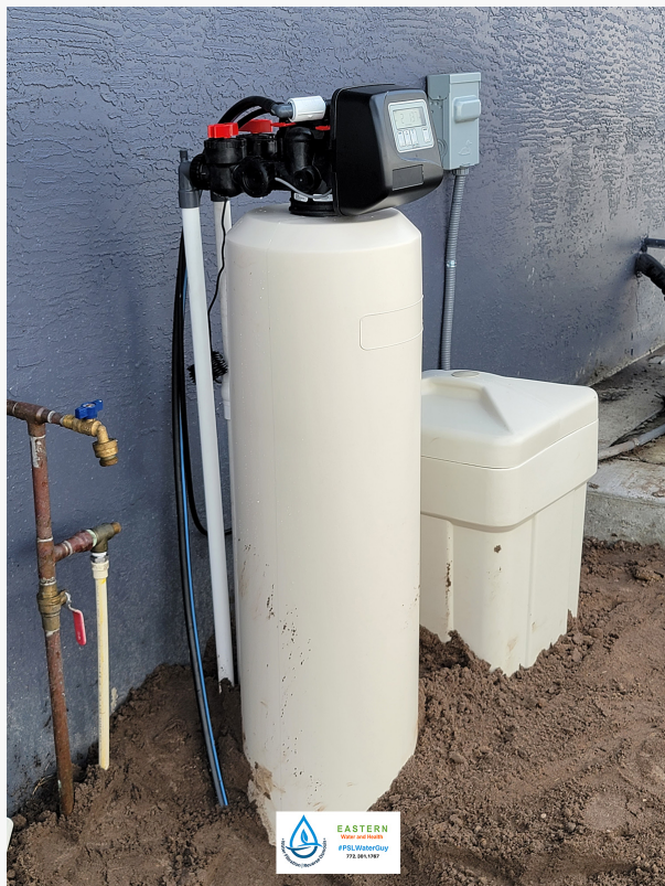
Water Softener System Installation Port St. Lucie
