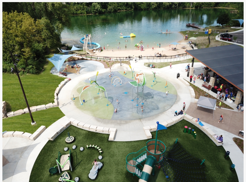
CRS designed park complete with Splashpad, playground, shade & shelter.
