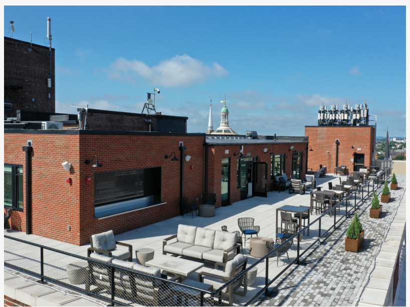
Yorktowne Hotel in York, PA. - newly renovated with a lightning protection system.
