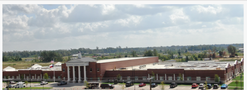
ILTexas new building at Colony Ridge Communities
