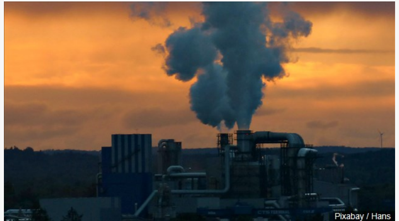
Coal Gasification Technology Market
