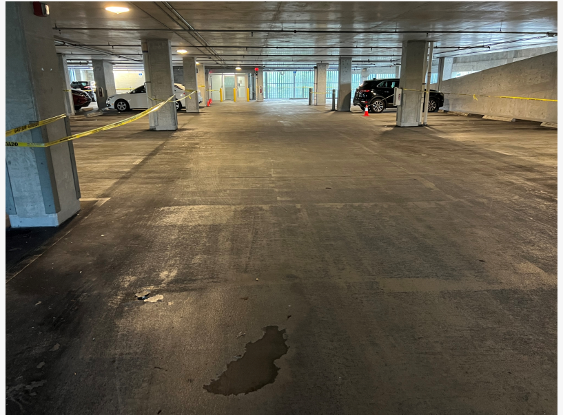
AC Marriott Parking Garage Before Waterproofing
