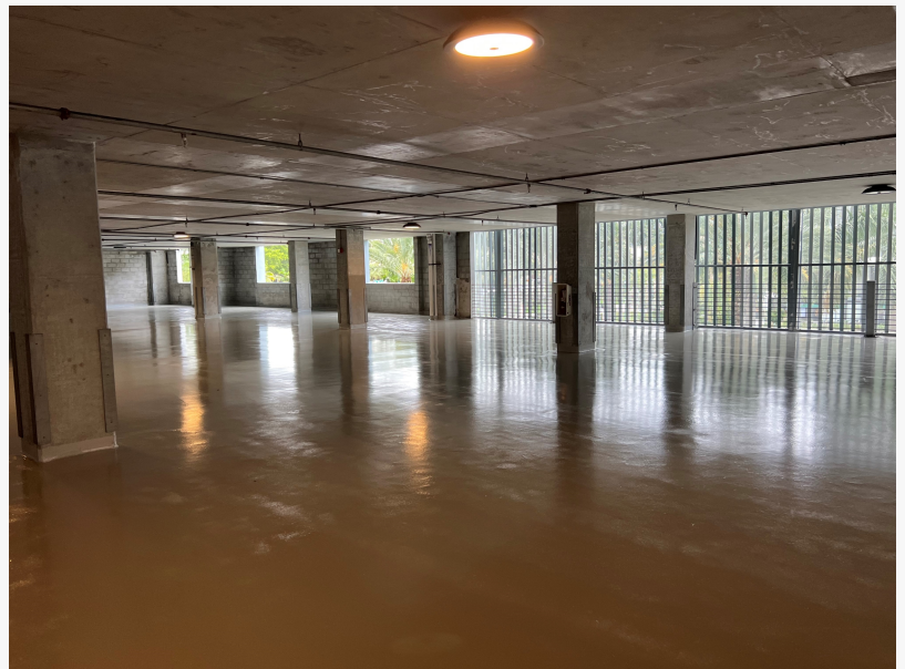
Completed AC Marriott Parking Garage Waterproofing Project
