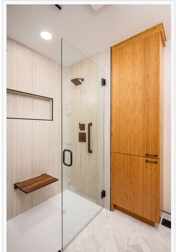
Remodeled ADA accessible guest bathroom with zero-entry curbless shower and custom grab bars.
