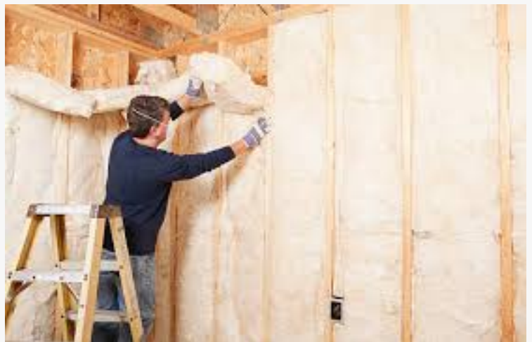
Tax Credit for Attic, Wall and Crawl Space Insulation
