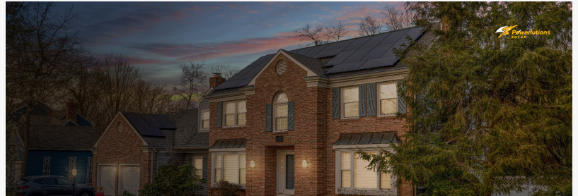
Beautiful house with solar panels.
