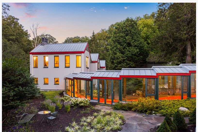
Water Run | Hudson Highland Estate
