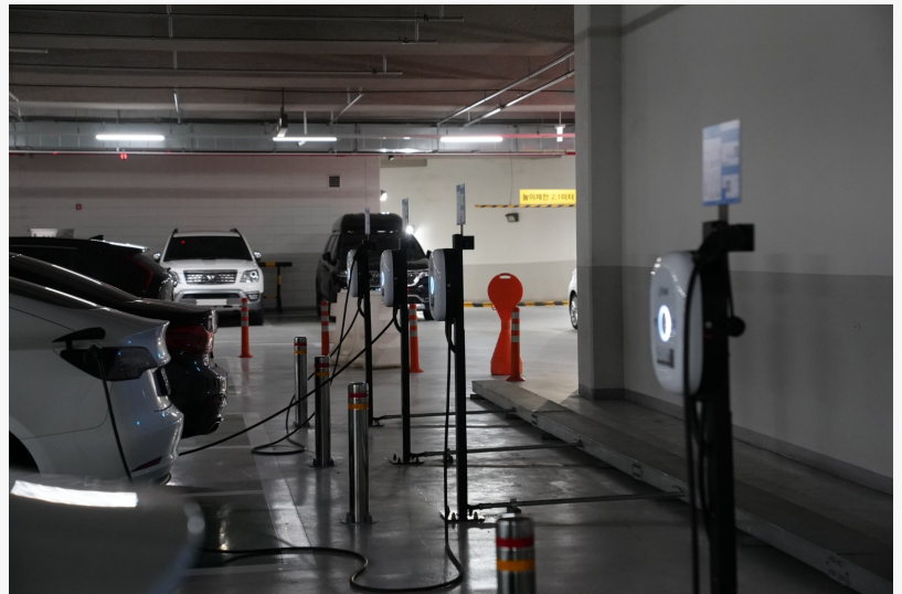
EVAR's charging solution installed in the parking lot of the Gyeonggi Business Growth Center (Photo = beSUCCESS)
