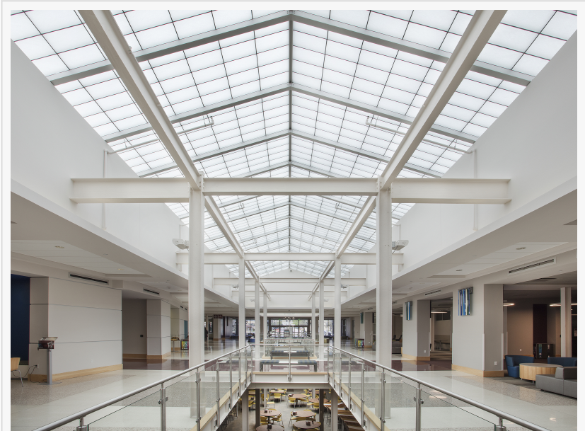
GridSpan Fiberglass Roof System (formerly known as Guardian 275 Skylights) at Texas A&M University Commons in College Station, Texas
