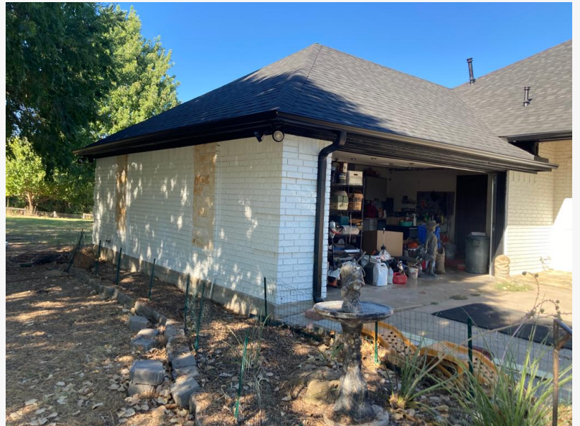
Gutter Company Fort Worth
