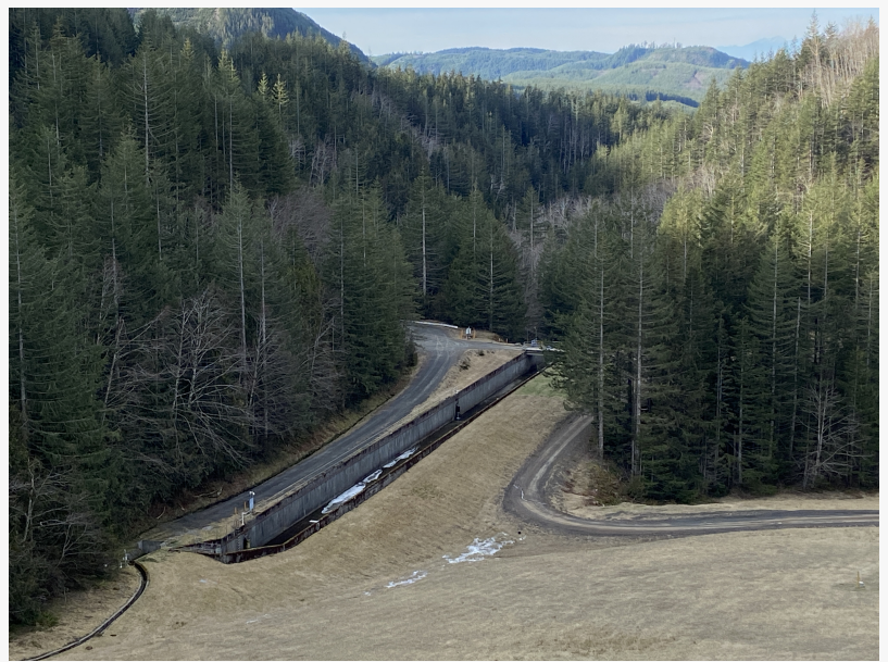
South Fork Tolt Spillway Options Analysis Project
