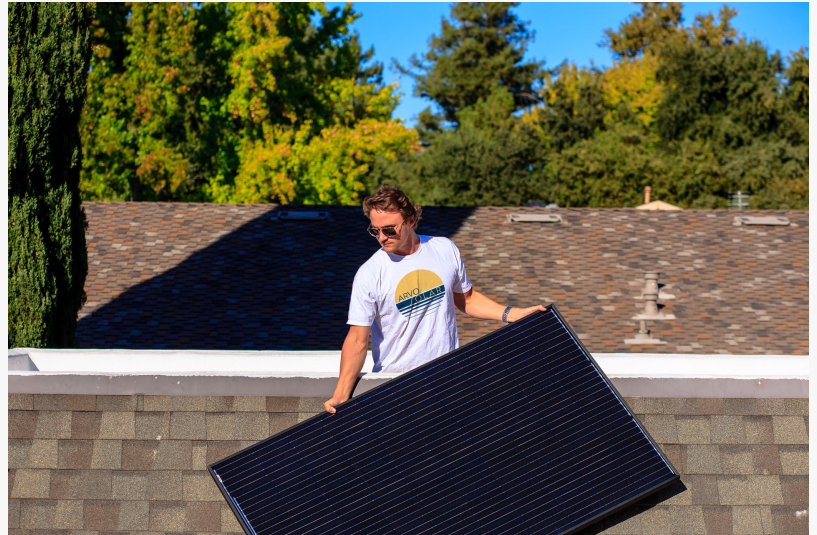
Arvo Solar team member installs solar panel.
