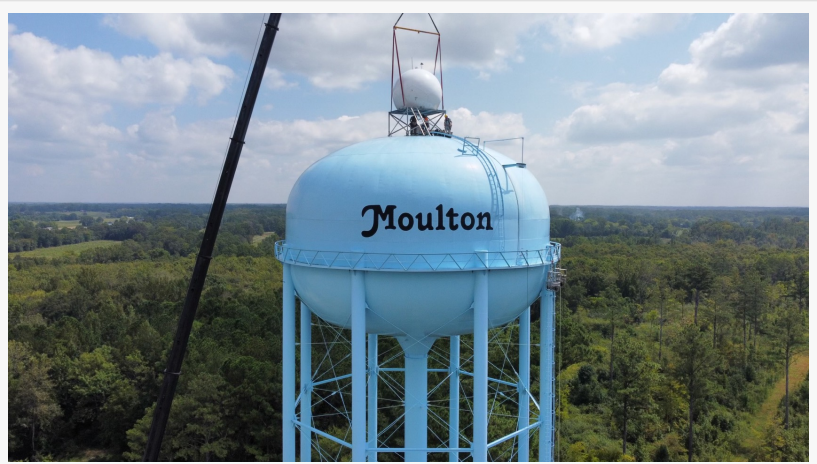
Crews lift Moulton radar into position
