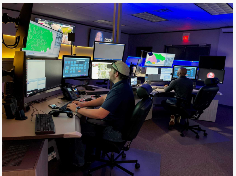
Texas Emergency Communications Center is located in Spring, Texas
