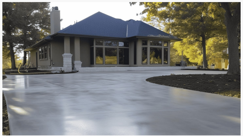
A freshly poured concrete driveway. Featuring a smooth finish, designed and installed by Core Concrete Contractors
