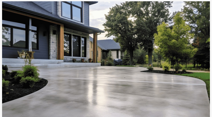
A recently poured and finished concrete driveway installed by Core Concrete Contractors in Champaign, IL.
